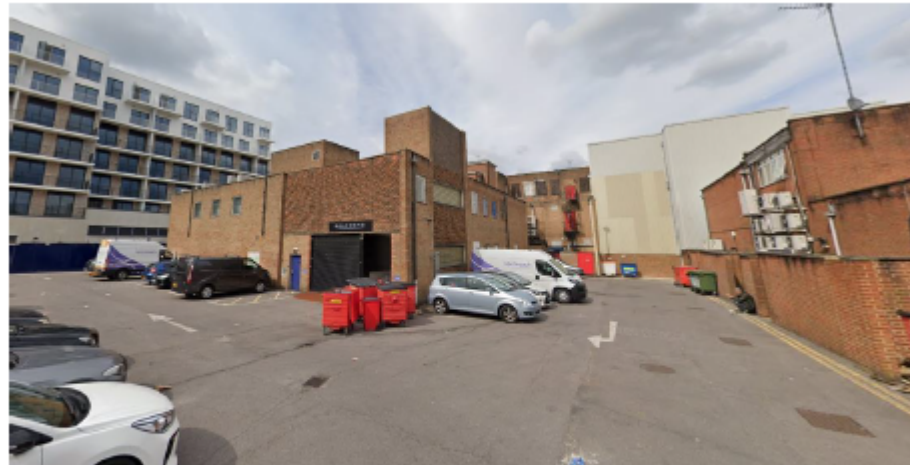
Photographs from September 2020 of rear part of nos. 32-34 Queens Square which are proposed to be locally listed for their historic and aesthetic value
