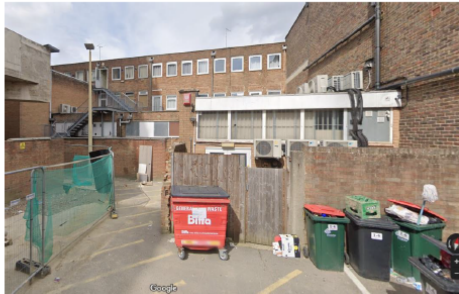
Photographs from September 2020 of rear part of nos. 30-40 Queens Square which are proposed to be locally listed for their historic and aesthetic value
